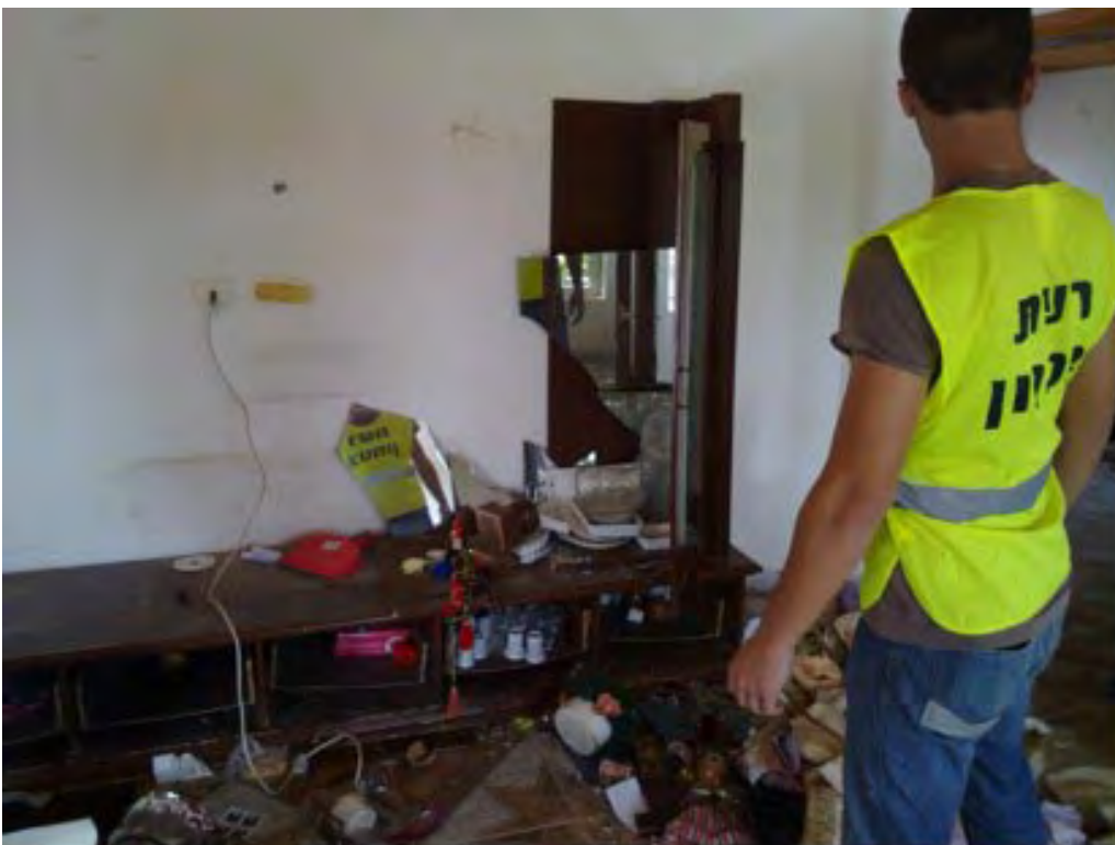
Figure 7.2: According to residents, the youth vandalized homes (Photos by Ata Abu Madyam, Arab Negev News )
